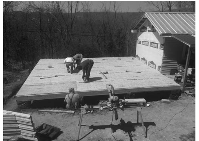
Awesome progress being made on the Carrs' addition
